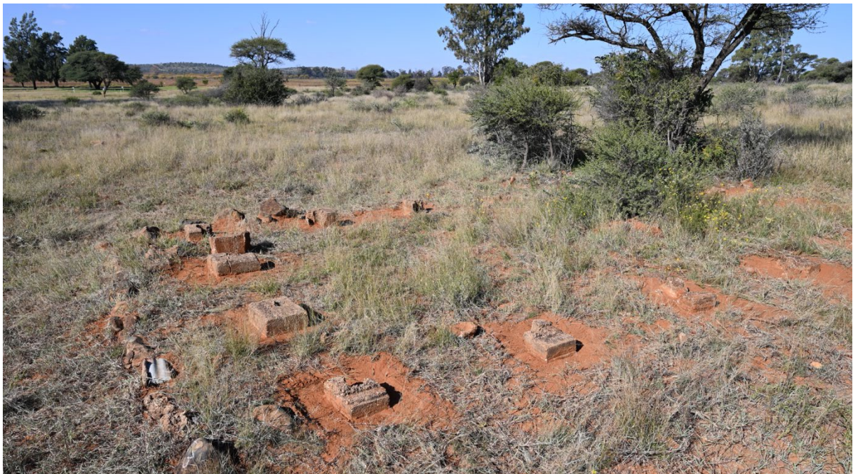
Fig. 4. Exposed foundations of one of the two hundred bungalows that provided accommodation for a group of six internees (photo by J. Hasil).
