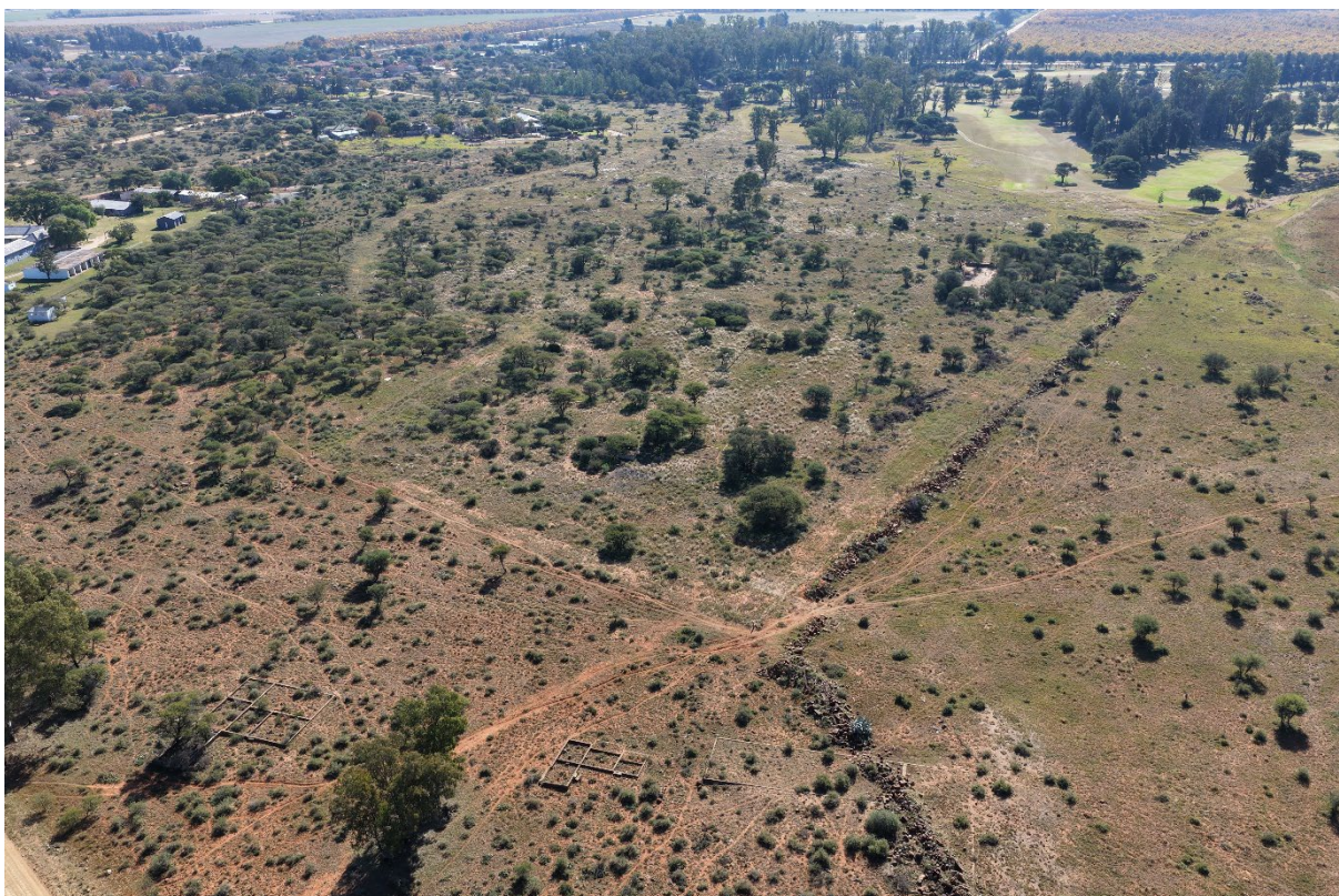
Fig. 1. Camp Andalusia, general view. In the foreground, the foundations of buildings used by the guard detachment are clearly visible (photo by P. Hasil).
